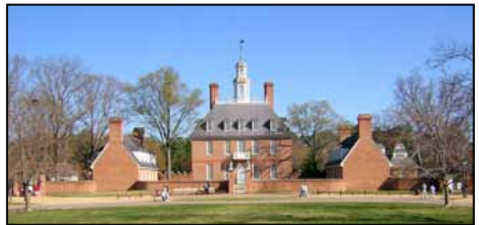
Governor's Palace Gov. Jefferson's residence in Williamsburg
